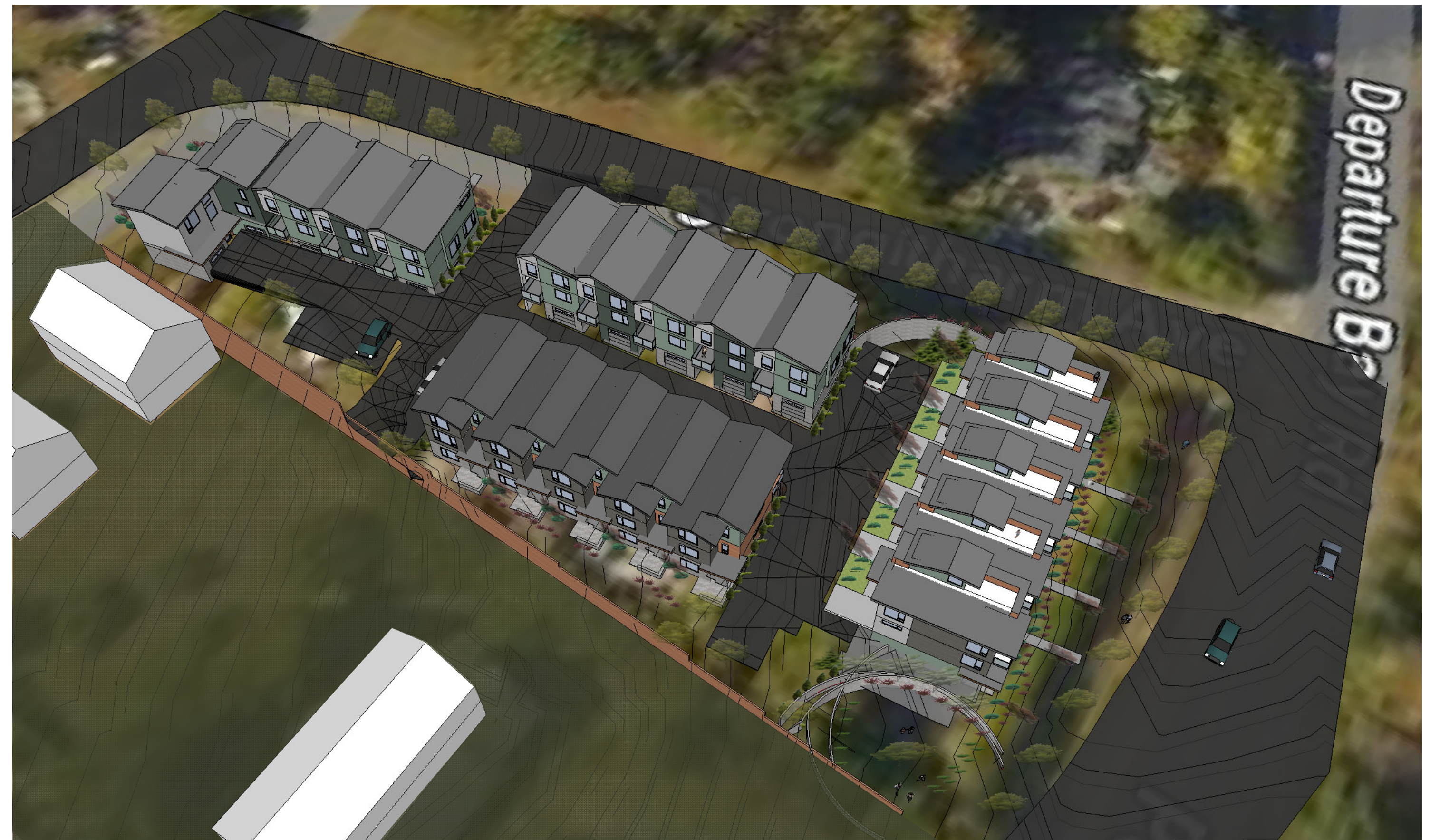
AERIAL VIEW FROM DEPARTURE BAY ROAD
